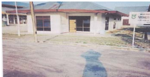
Figure 2. Office of fish landing Dumai
