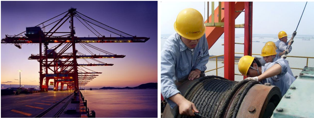
Figure 1. A steel rope renewal activity in the container terminal
